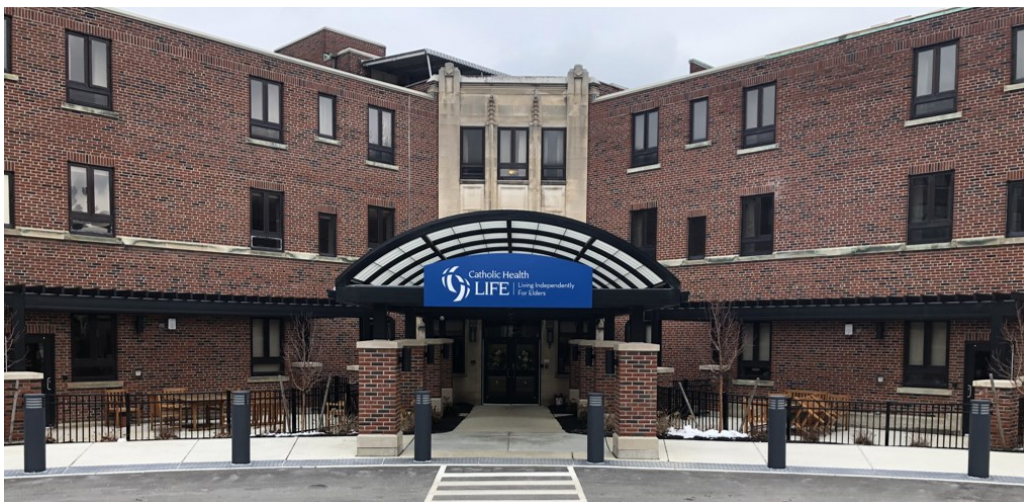
St. Francis Residence, Buffalo, NY, became home to the Catholic Health Programs of All-inclusive Care for the Elderly (PACE), serving the residents of Buffalo while also allowing the sisters to receive health care without leaving home. (Photo used with permission)
